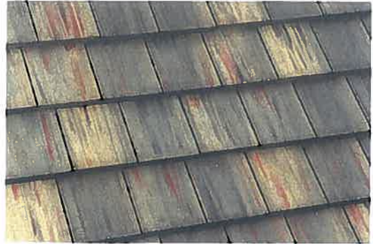
FLAT SMOOTH ROOF EAGLE 4634
